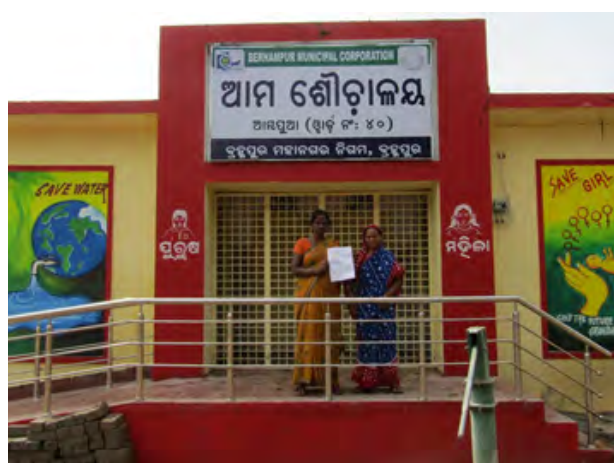
Figure 49- Work Order and Key for CT at Ambapura Crematorium ground given to Sri Sri Maa Jagadamba SHG
